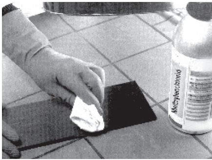
Figure 13: Chemical treatment of a previously sanded surface
