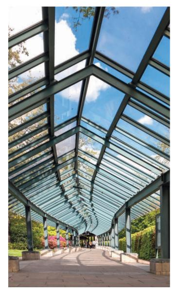
Thermal processes are ideal for forming glazing to the required shape. PLEXIGLAS® can also be cold-curved. That makes it possible to realize individual design ideas in public spaces at no great expense. From curved roofs for bus stops to barrel vaults above a hotel entrance, a welcoming exterior makes for a pleasant atmosphere. Experience also shows that attractive structures are less likely to be vandalized.
